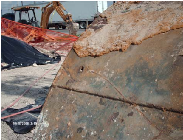
Old steel tank being removed
