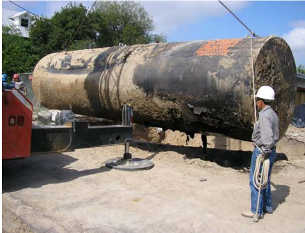
Old steel tank being removed
