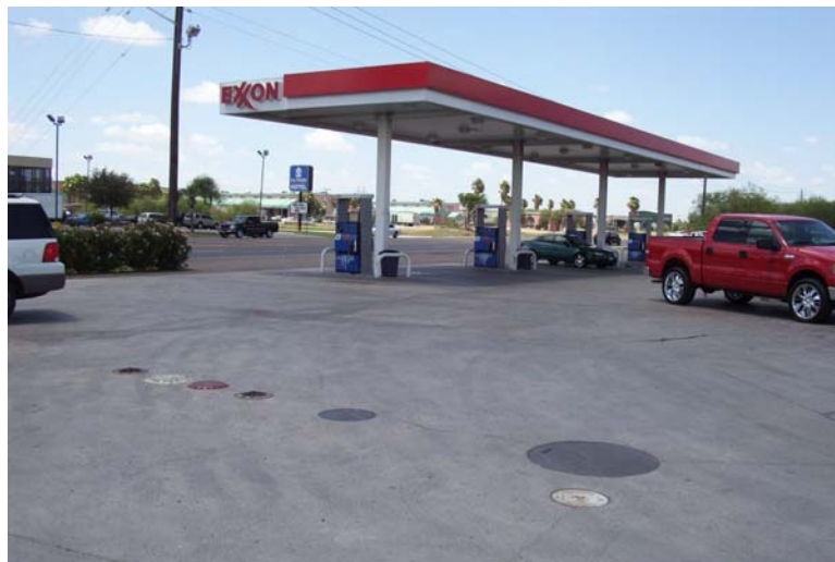
Typical auto fueling area with gas and diesel for smaller trucks
