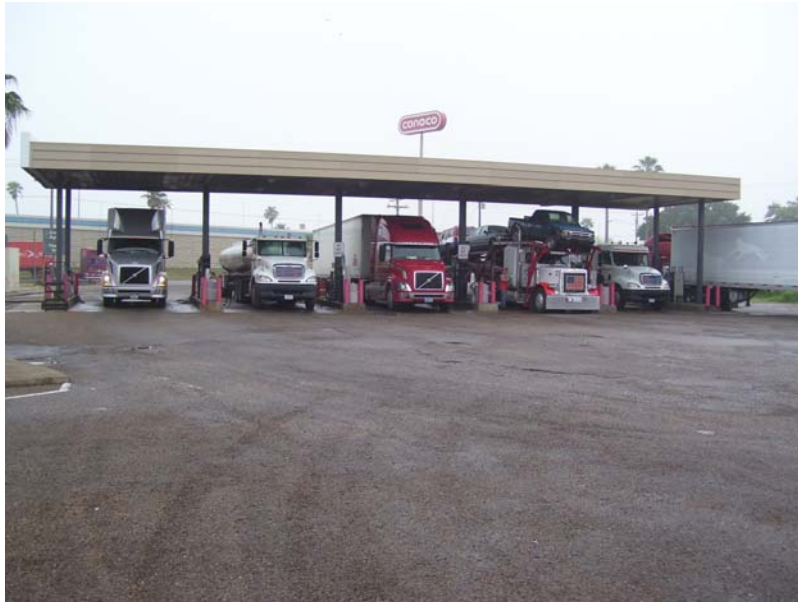
Truck fueling area
